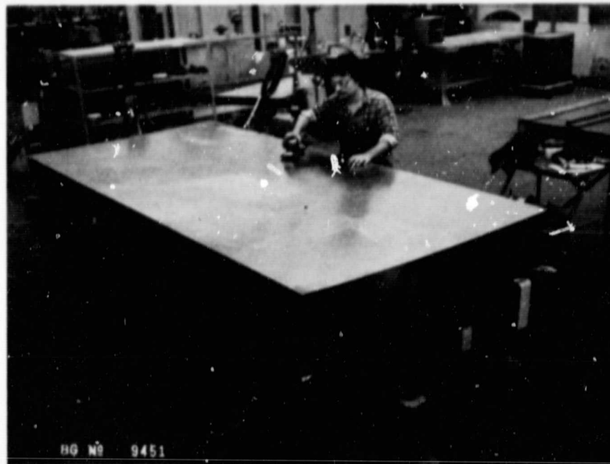
Figure 2-50. Completed Cover Bonding Tool for 100-Inch Subcomponent
