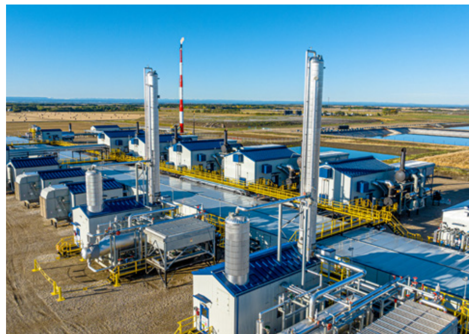
Pipestone North 16-28-71-9W6 facility
