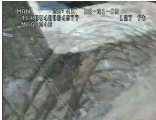
Figure 2: An example of powerlines (lower left, diagonal) as a danger in exterior structural inspection.
