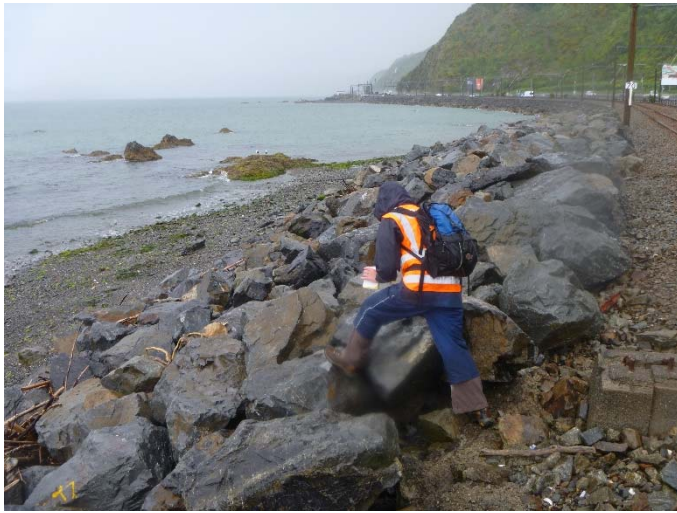
Photo 7: Rock stack in sub-tidal edge
