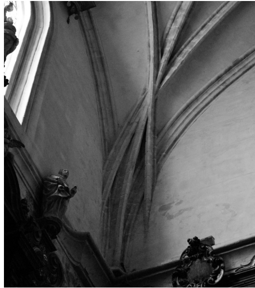
Fig. 8: Springing of the vault.
