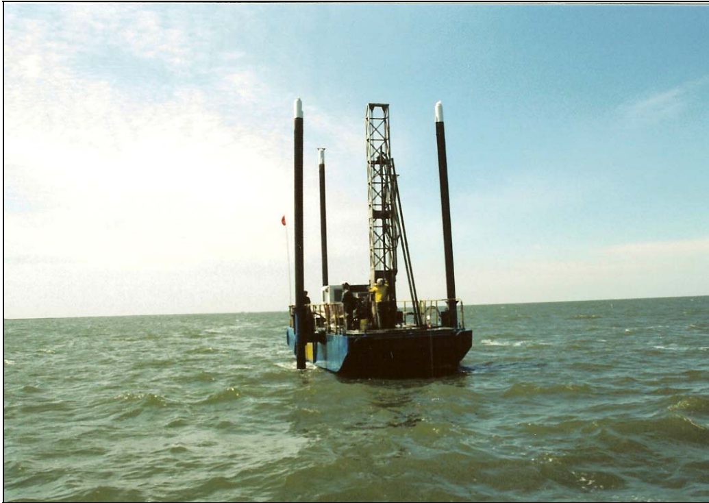
Jack-up drill drilling in open waters
