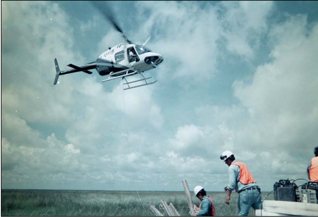
Helicopter picking up equipment from a flatboat
