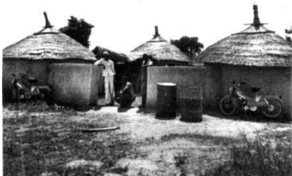
ICRISAT buildings used by economics program investigators in a village in Upper Volta.
