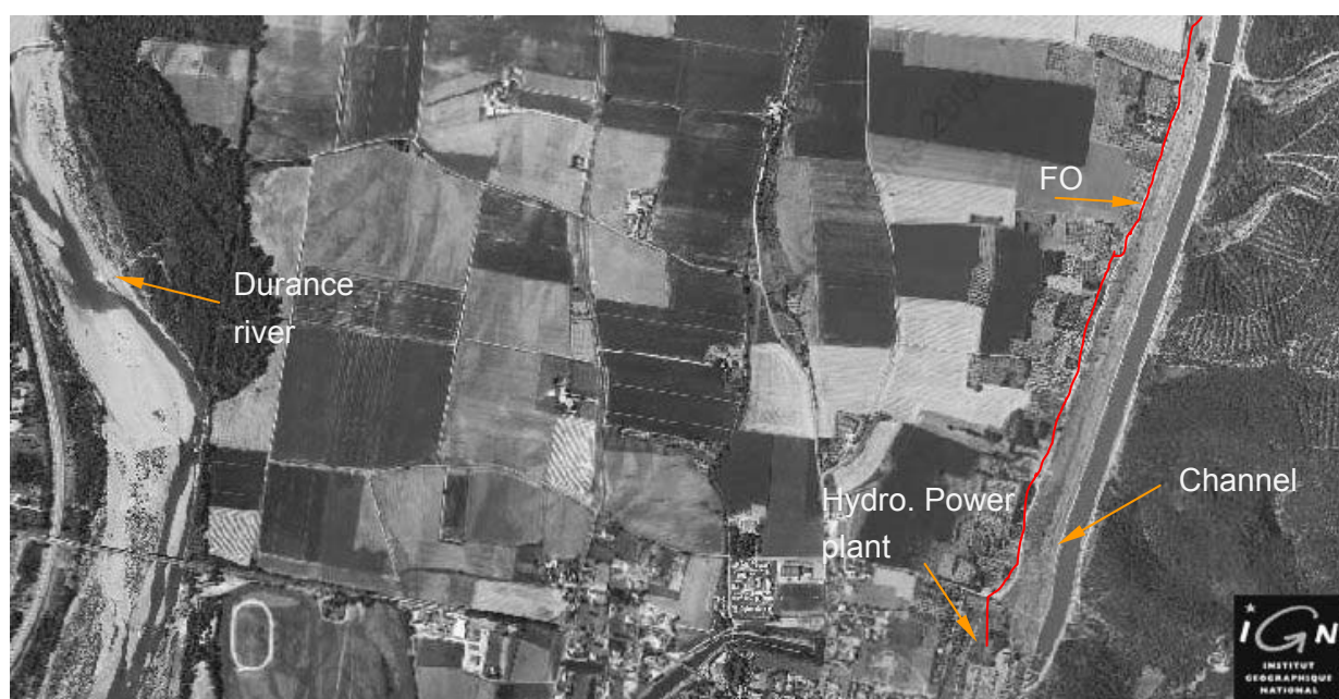
Figure 1: Aerial view of Oraison canal
