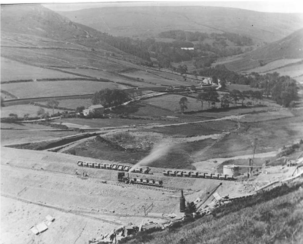
Figure 3: Fill placed on shoulder of the dam by side tipping from railway wagons
