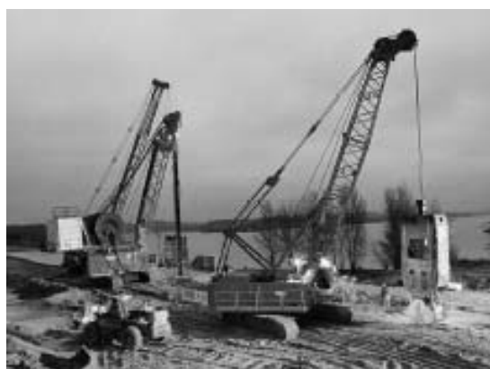
Figure 7: Cut-off of La Ganguise dam
