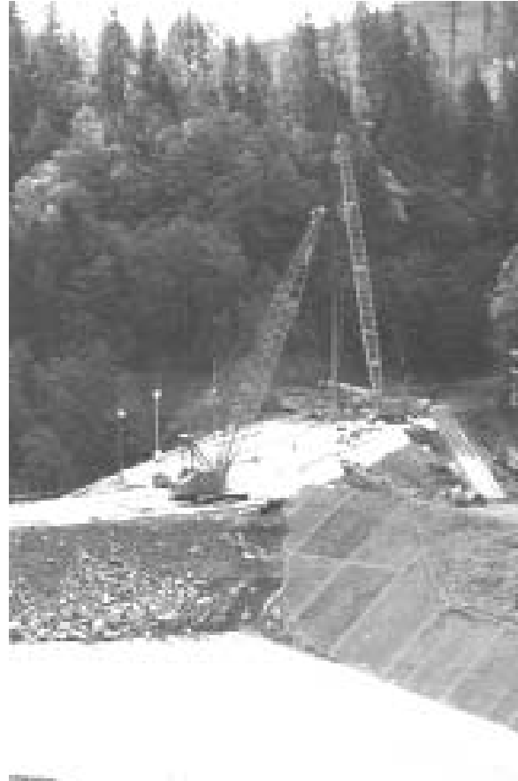
Figure 8: 120m diaphragm wall of Mud mountain dam
