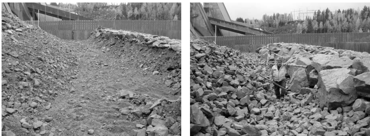
Figure 9: Foundation of the toe-berm
