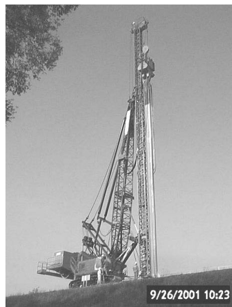
Figure1: vib wall under construction
