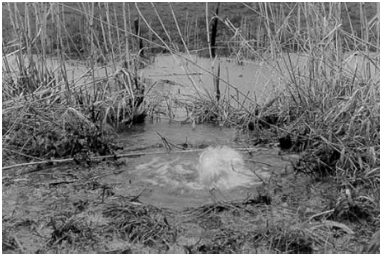
Figure 2: Sand boil behind a river embankment.
