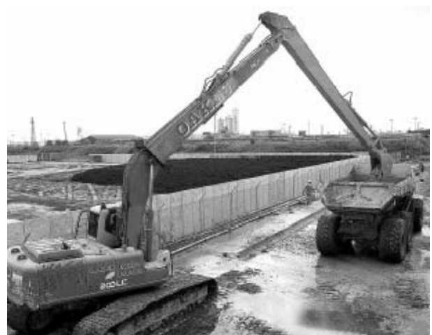
Figure 4: trench excavated by backhoe
