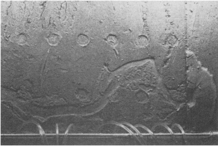
Figure 5: Result of piping test showing erosion pattern [Wit, de et al, 1981]
