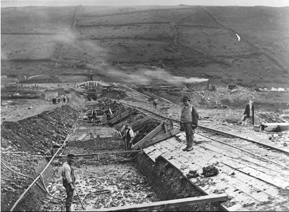
Figure 1: Puddled clay fill placed in cut-off trench up to level of dam foundation
