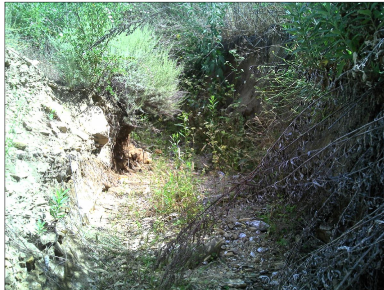
Photograph 3: Drainage A near mid-point of on-site channel looking downstream/south.
