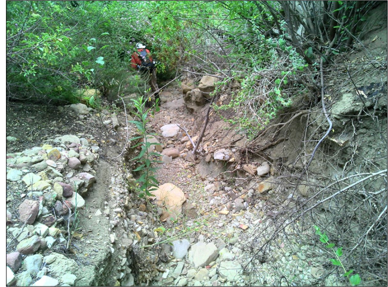
Photograph 2: Upper Drainage A near eastern site boundary looking downstream/southeast.
