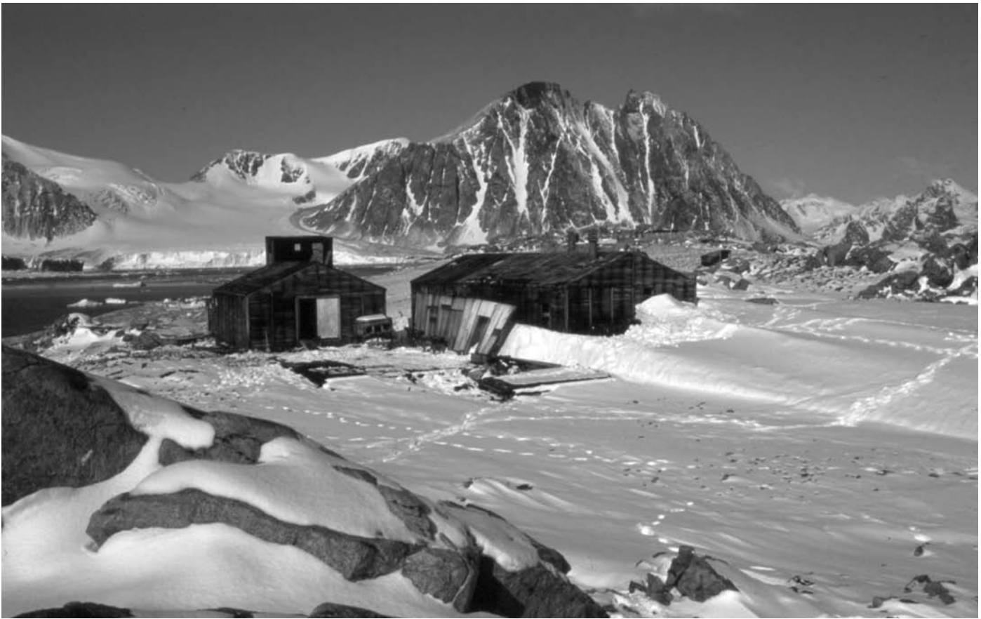
FIGURE 3. The abandoned East Base on Stonington Island, Antarctica. The Science Building with its weather tower and the Bunkhouse building were intact. The crate containing a spare engine for the Curtis Wright Condor biplane can be seen in front of the Science Building. (Photo by Noel Broadbent, 1992)
