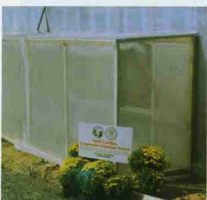
AA. Screening structure retrofitted to a commercial greenhouse.
