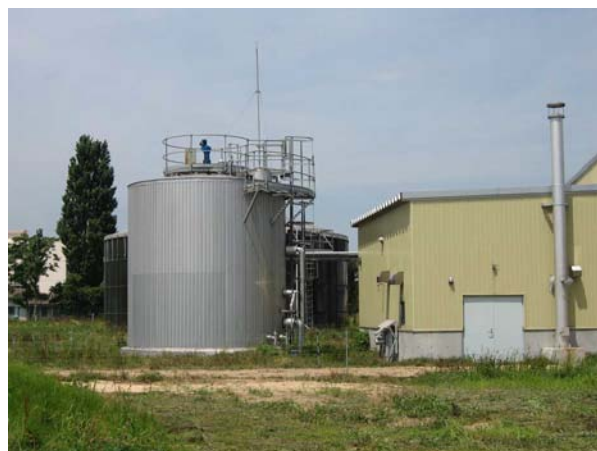
Fig. 4-31. Biogas system with methane fermentation.
