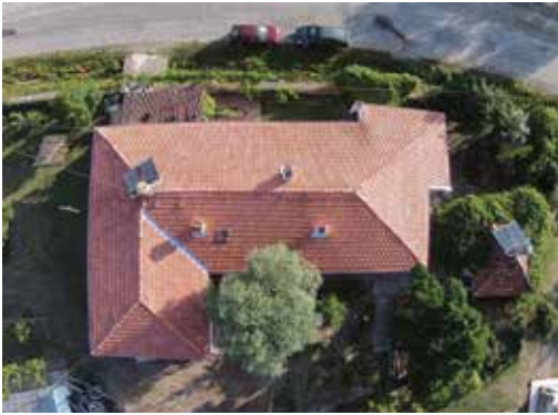
Figure 14. The new roof on the excavation house
