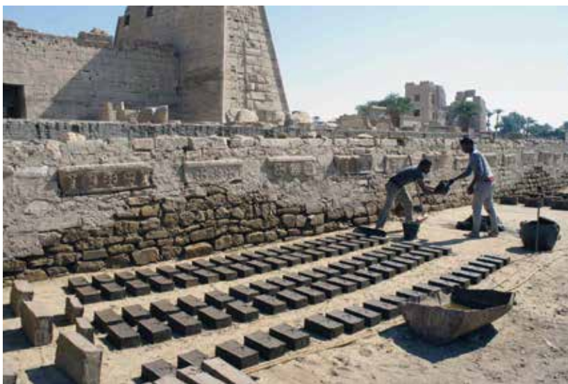
Figure 1. Chicago House workmen manufacturing new mudbricks for restoration. Medinet Habu (photo: Ray Johnson)
