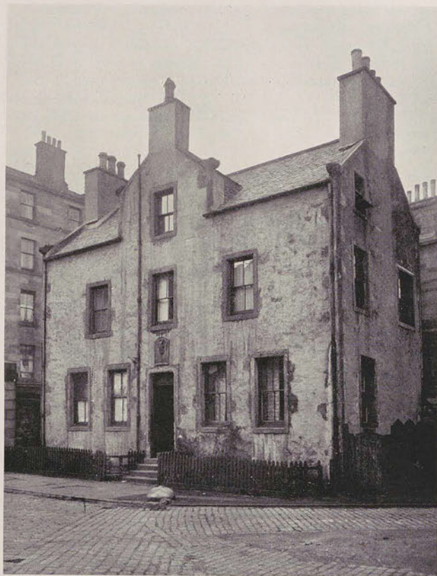
OLD HOUSE AT ST. LEONARDS COAL DEPOT
