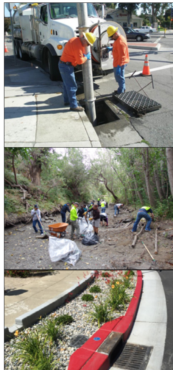
Crews vacuum stormdrain to remove contaminants, and volunteers remove trash from creek. Green infrastructure in nearby Palo Alto showcases how urban land use changes can benefit water quality and reduce street flooding. Photos: SCVURPPP and City of San Jose
