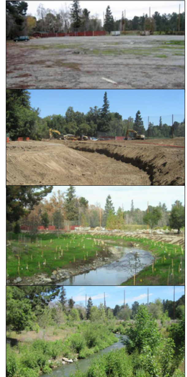
The transformation of a stretch of Stevens Creek at Blackberry Farm near Cupertino, from parking lot in 2008 to thriving riparian corridor today. Photos: City of Cupertino
