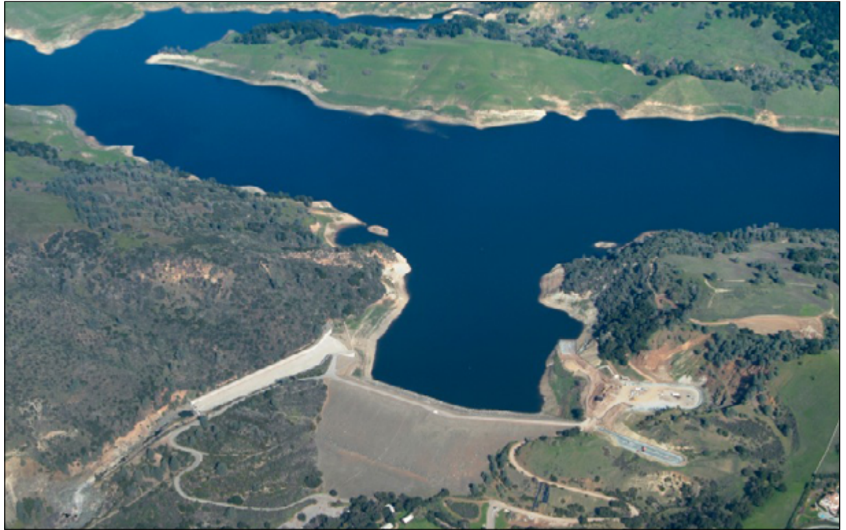
The District's Anderson Dam in the Coyote Creek watershed, built in the 1950s in a natural gorge east of Morgan Hill, is now undergoing a seismic upgrade. Photo: SCVWD
