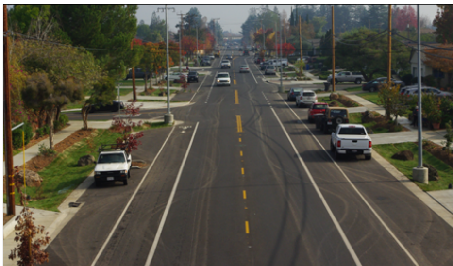
Hacienda Avenue, Campbell, before (top) and after (bottom) green infrastructure improvements, including bioretention basins along sidewalks which provide stormwater management benefits. Photos: SCVURPPP
