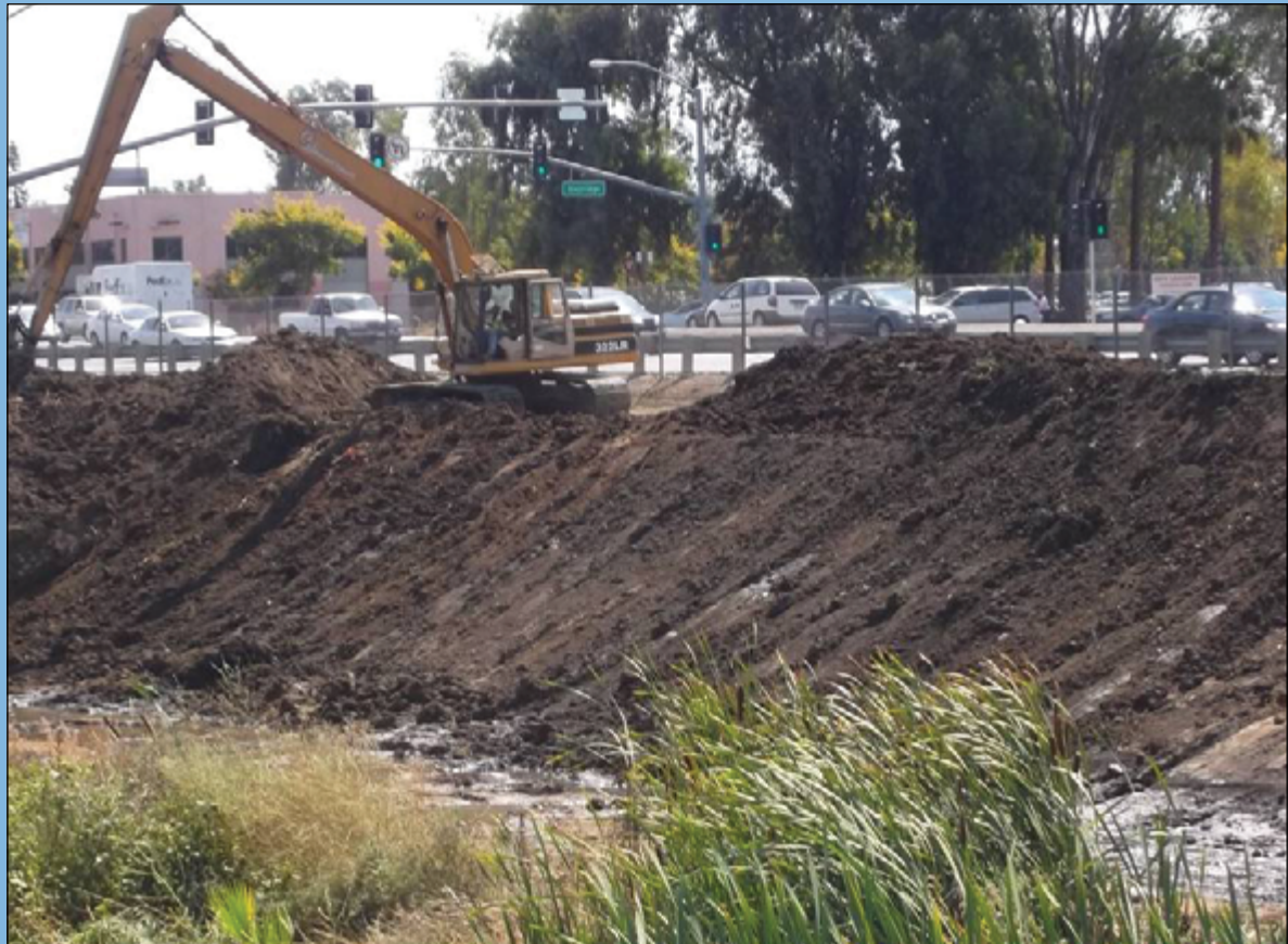
Removing sediment from Thompson Creek, San José, to maintain stream capacity and condition. Photo: Valley Water
