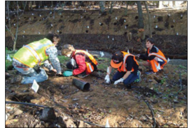
Kids help plant and restore the banks of Adobe Creek in Edith Park, Los Altos Hills.
