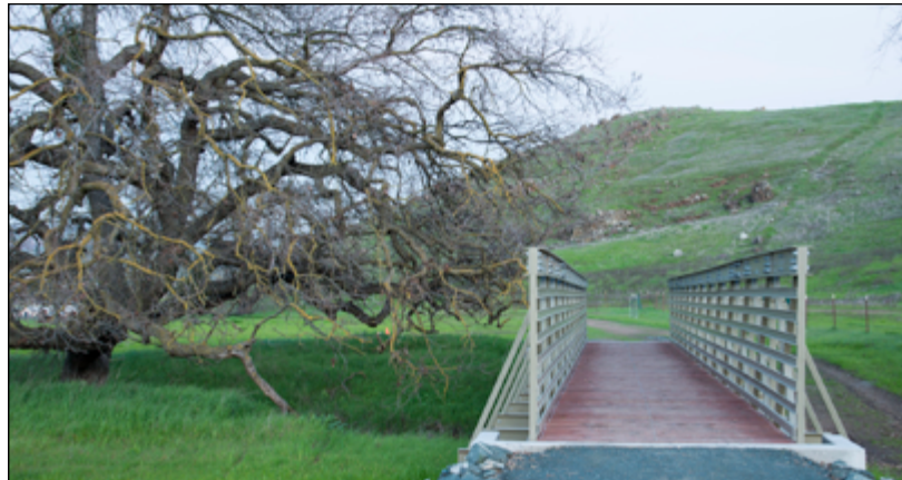
Trail bridge over Coyote Creek. Photo: Santa Clara Valley Open Space Authority
