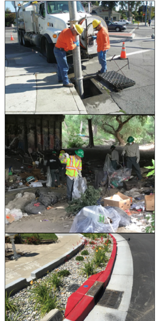
Crews vacuum stormdrain to remove contaminants, and volunteers remove trash from creek. Green infrastructure in nearby Palo Alto showcases how urban land use changes can benefit water quality and reduce street flooding. Photos: SCVURPPP and City of San José
