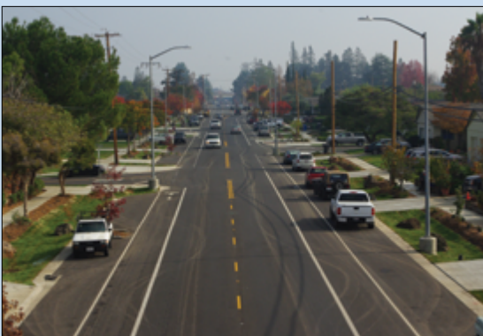
Stormwater improvements to Hacienda Avenue in Campbell.
