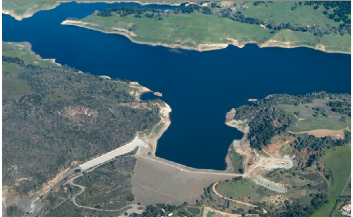
Valley Water's Anderson Dam in the Coyote Creek watershed, built in the 1950s in a natural gorge east of Morgan Hill, is now undergoing a seismic upgrade. Photo: Valley Water
