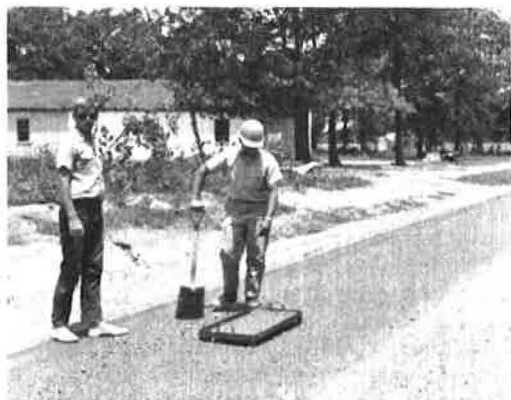
Figure 1. Tray for sampling surface treatment aggregate as used.
