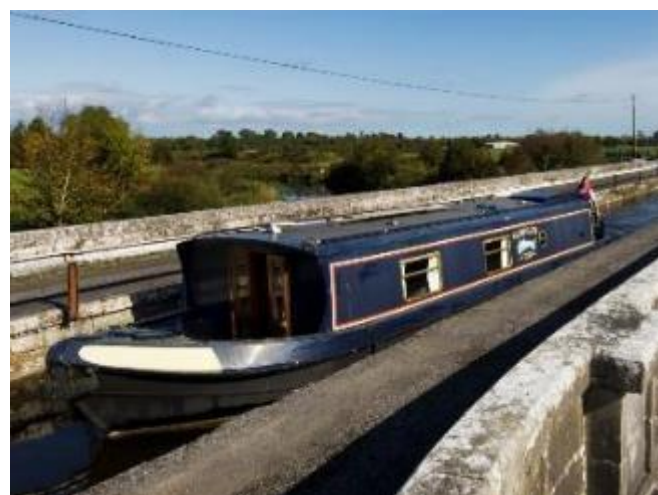
Whitworth Aqueduct, Royal Canal
