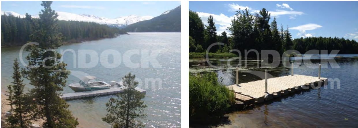
Examples of modular floating docks used by Parks Canada in a marine park (left) and an eastern lake based park (right).
