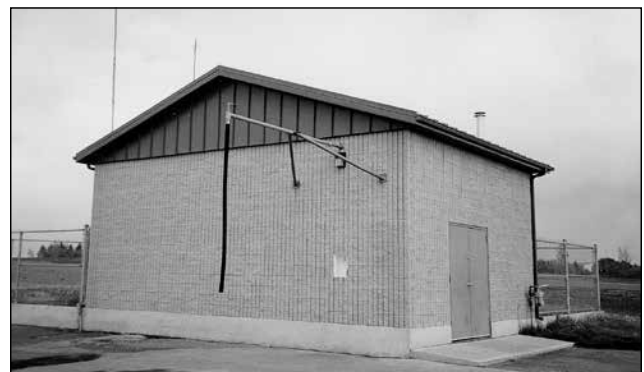
Figure 5. Tank loading facilities
