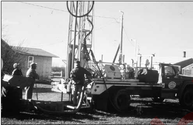
Figure 6. Test drilling to locate groundwater aquifers
