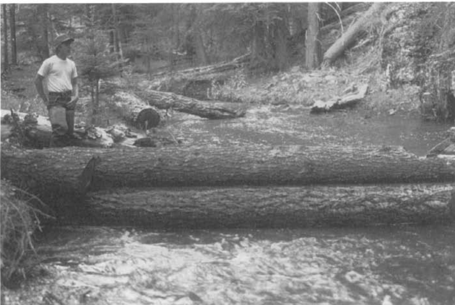
Fig. 14-1. Single (A) and multiple (B) log stream-improvement structures in McKnight Creek, New Mexico. Photograph by J. N. Rinne, August 1977.
