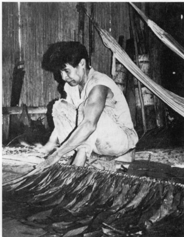
Carijona man preparing a roof covering
