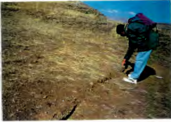
Plate 5.7a Surface crack at Mapeleng.
