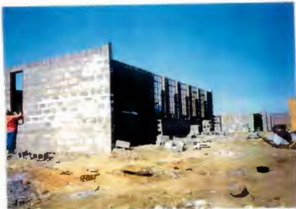
Plate 5.10c Community hall under construction
