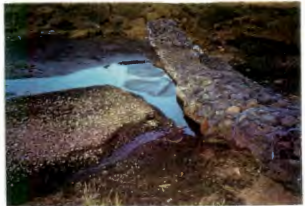
Plate 5.4b Gabions to control erosion in the Bokong wetland.
