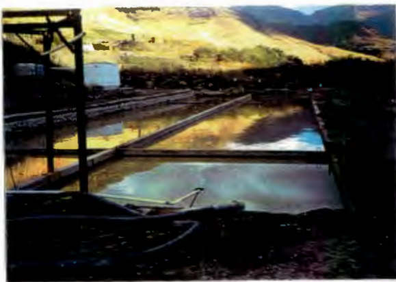
Plate 5.6i Settling ponds to treat effluent before depositing into the stream.
