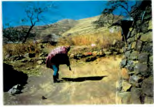
Plate 5.7b Surface crack through the village.
