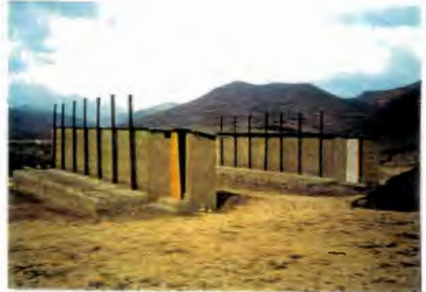
Plate 5.10b Sanitary facilities in local Schools.
