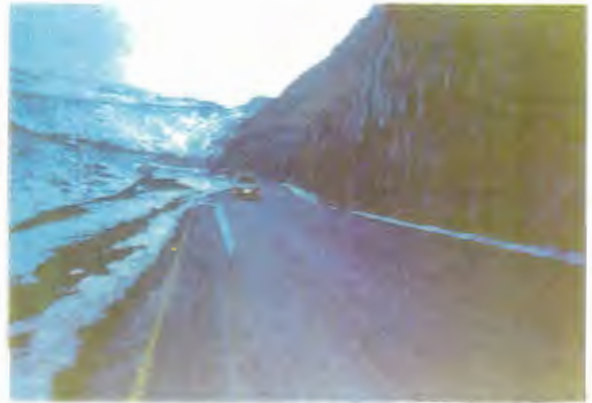
Plate 5.3b All weather access road to the highlands of Lesotho.
