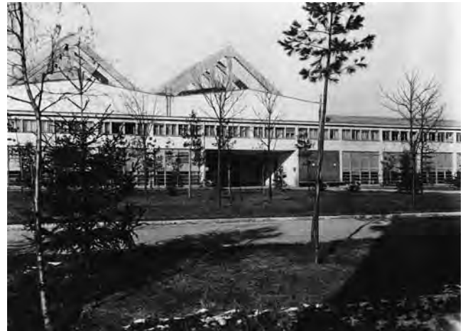
Fig. 3: The Litoštroj factory was a large-scale industrial plant, designed as an open structure in green surroundings, with innovative building structures to present the enforcement of the new society in industrial development. The metalworking plant has a suspended roof fixed on triangular brackets. Architect: Miroslav Gregorič, 1946
