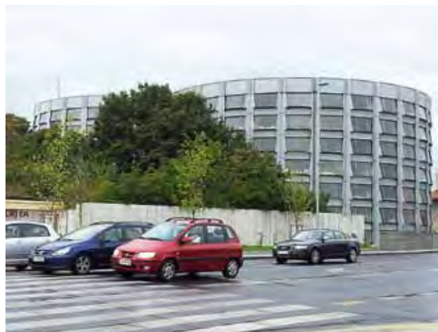
Fig. 11: The Garage in Ljubljana showcases the architect's innovativeness in building technology and structure, which was constantly researched in the projects of Savin Sever, 1969
