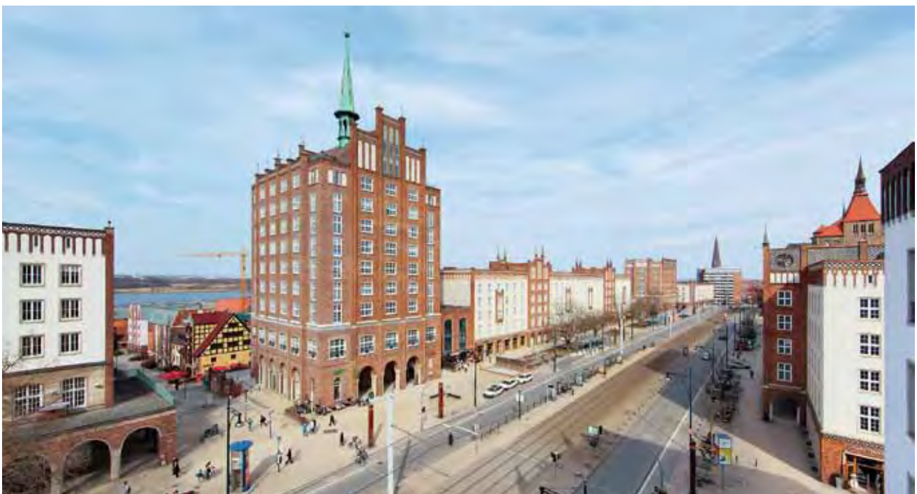
Fig. 1: Rostock, Lange Strasse, buildings on the north side, 2013
