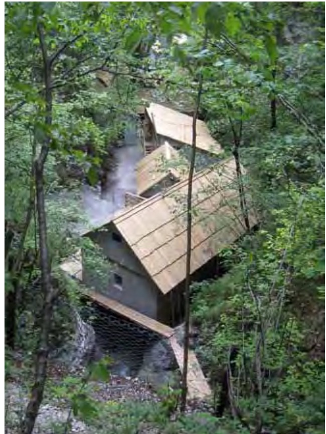
Fig. 1: Franja Partisan Hospital after reconstruction
