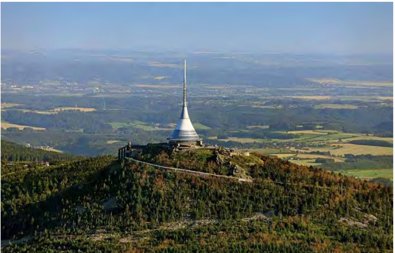
Ještěd mountain-top hotel and television transmitter. Its design was developed between 1963–66, construction itself took place from 1966–73. The tower's architect is ing. arch. Karel Hubáček (1924–2011), who was awarded the prestigious Auguste Perret Prize for his design by the International Union of Architects in 1969 Berghotel und Fernsehturm „Jeschken“. Die Anlage wurde 1963–1966 entworfen und zwischen 1966 und 1973 realisiert. Der Architekt Karel Hubáček (1924–2011) erhielt 1969 dafür den Auguste-Perret-Preis der Internationalen Vereinigung der Architekten (UIA)
