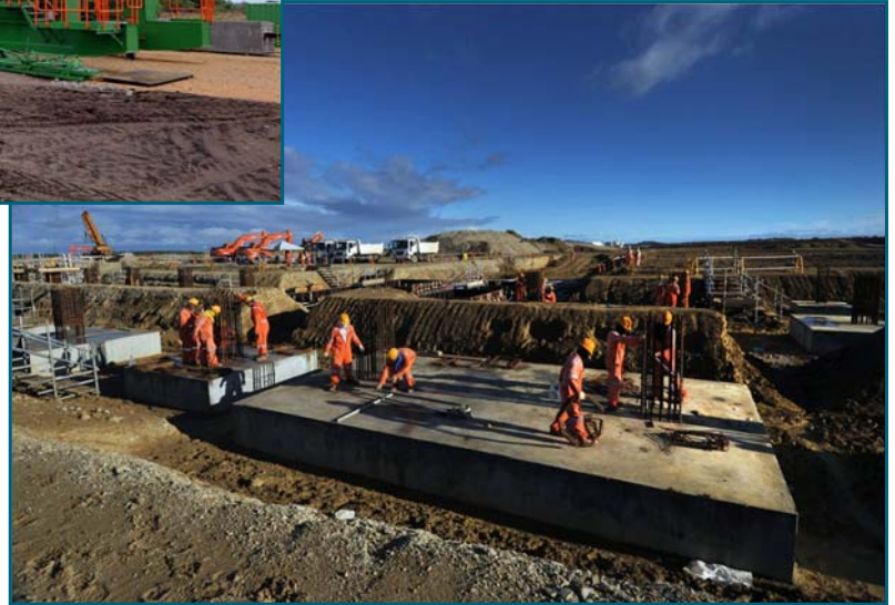
Process pipe rack construction
