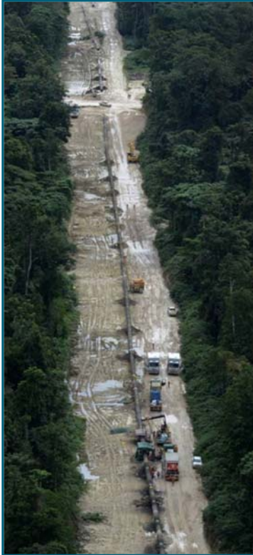
Pipeline stringing, onshore pipeline
