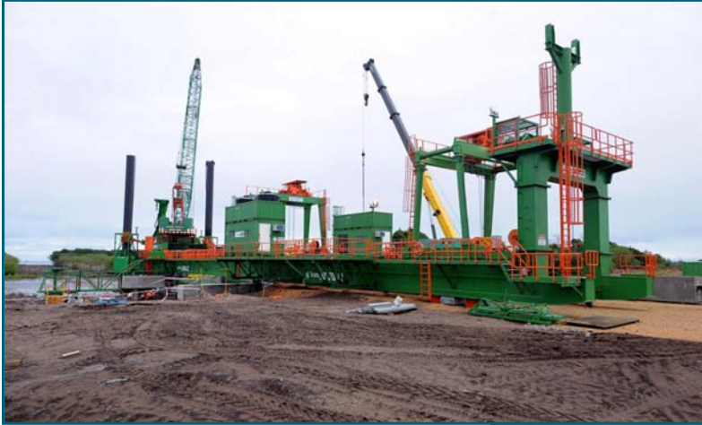
Marine jetty piling
