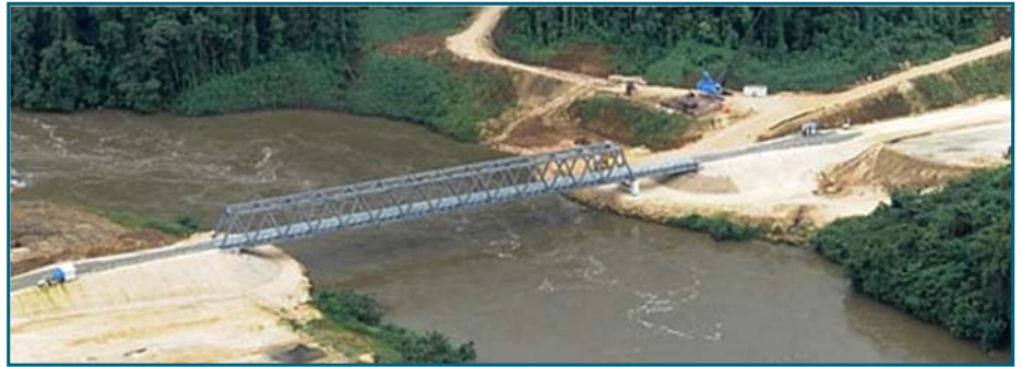
Completed Mubi River crossing
