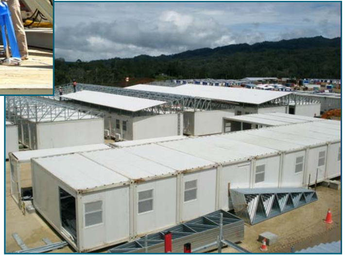
Hides Conditioning Plant - Pioneer camp construction
