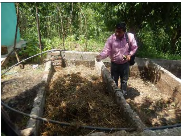
Compost Site Supported by Mid Himalayan Watershed Development Project, Mandi District (14 June 2017)
