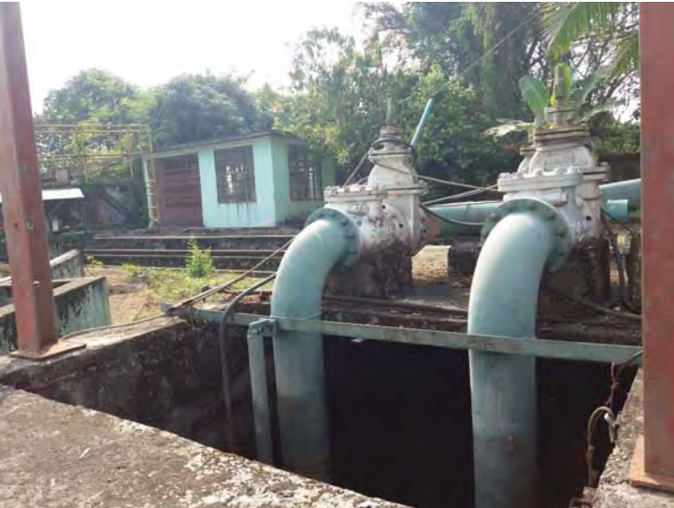
No.10 Return Sludge Pump Pit
