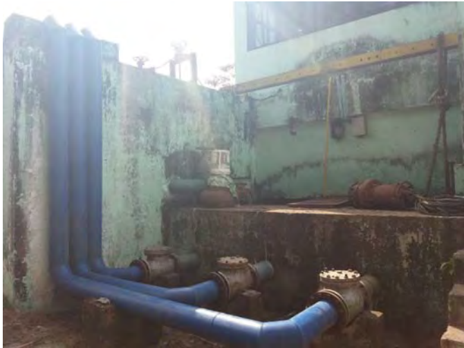
No.4 Pump Pit (Raw Water Pit)
