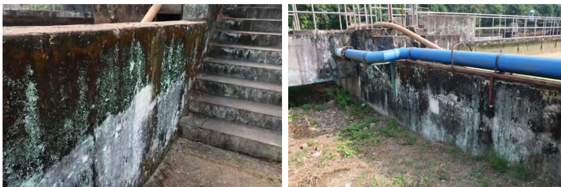
Photo 1: Concrete Surface of Reactor in C1 WWTP
