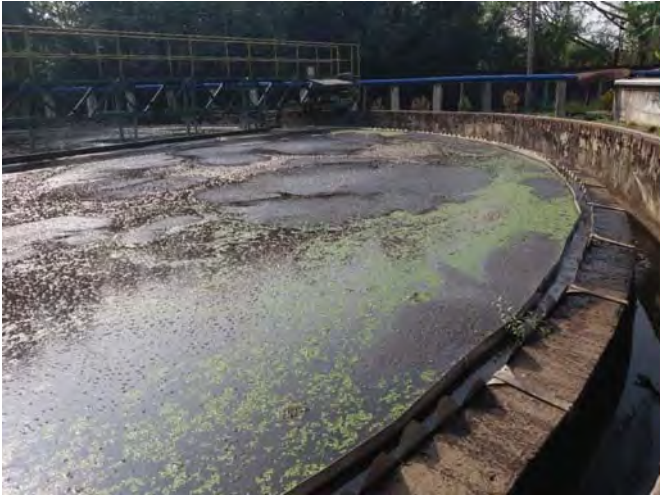
No.9 Secondary Settling Tank
