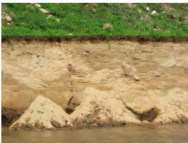
Figure 5-19 Exposed Sand Layer of the Dry River Bed
