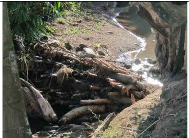
Private check dam to keep water for paddy (26. Oct. 2012, Houay Khing village)
