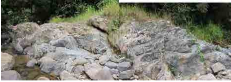
Photo 0-12 Outcrop of Numbuonamboto volcanic conglomerates on the left bank just beneath the powerhouse site
