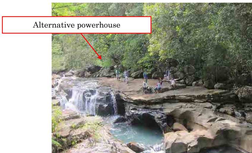
(Photo-2) Condition of alternative powerhouse site, which is the downstream of original intake site Geological condition is that bedding plane inclines gently to the upstream direction. (View from downstream of right bank (Nabiaurua Creek))
