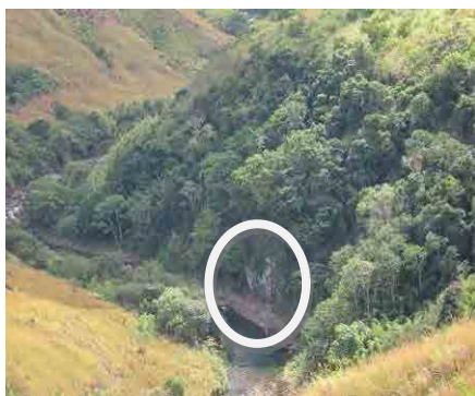
Photo 0-2 outlet of the Connection tunnel
