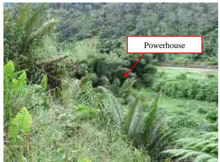
Photo-6 Condition of alternative powerhouse (View from the road to Waivaka village)
