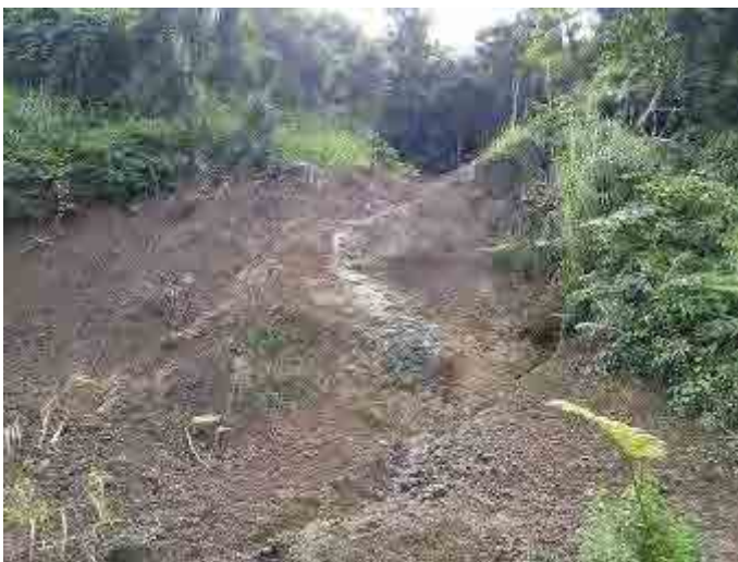
Photo-5 Condition of landslide near the penstock
