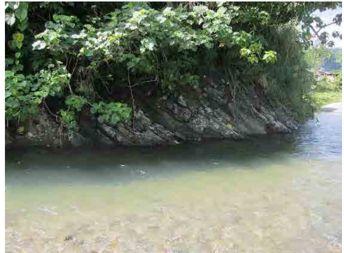
Photo-4 Outcrop of well-bedded mudstone and fine-grained sandstone on the left abutment of the weir site.
