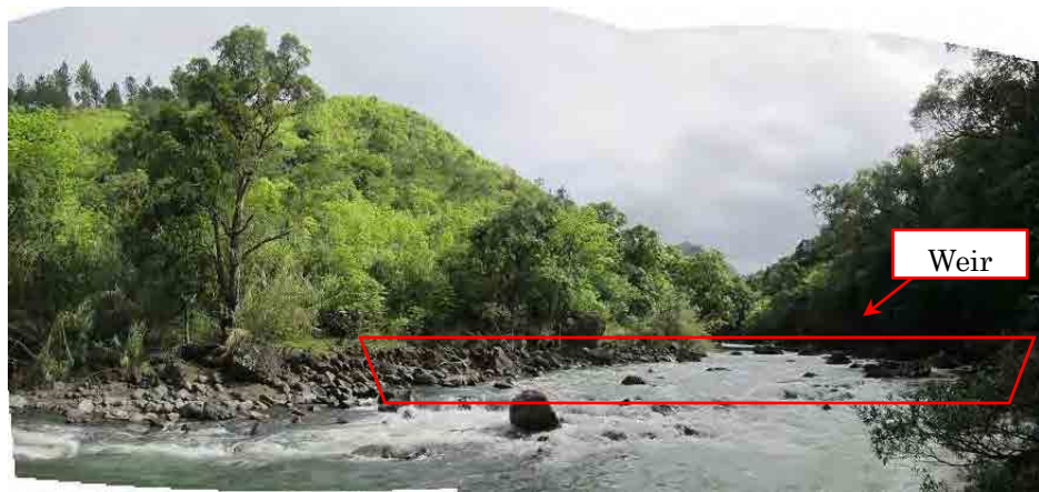
(Photo-1) Condition of original No.1 intake site
