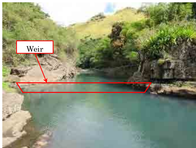
(Photo-6) Condition of weir of proposed No.7 downstream power station utilizing the head between the confluence and Nadarivatu power station
