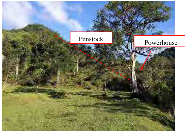
Photo-2 Condition of alternative penstock and powerhouse (View from approach road)
