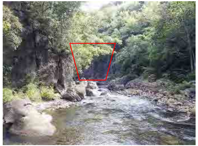
(Photo-3) Condition of alternative dam site for No.2 intake
