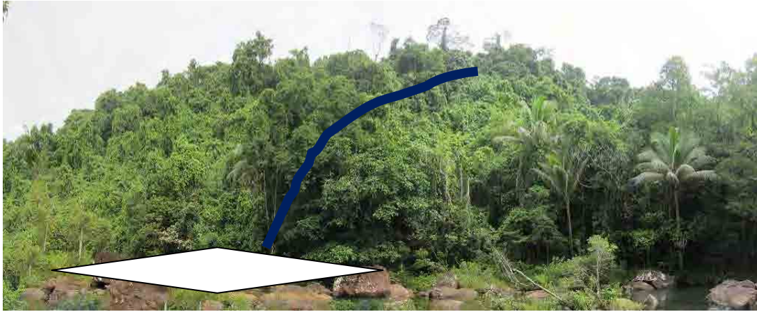
Photo 0-17 Planned Penstock line and the Powerhouse site which is on the right bank of Wailevu creek
