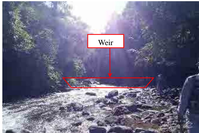
Photo-1 Condition of alternative weir Wairokodra River flow rate is about 1.5\text{m}^3/\text{s} . (View from upstream of Wairokodra River)
