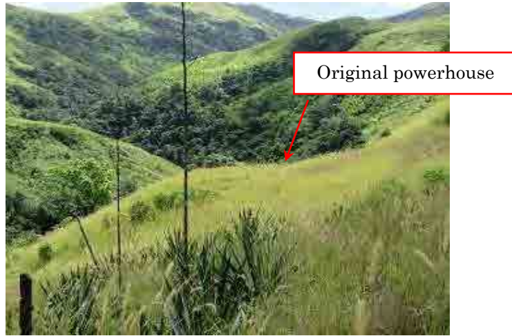
(Photo-6) Condition of original powerhouse (View from footpath on the way to original powerhouse)
