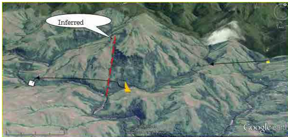
Figure 0-3 Whole view of the scheme on the GOOGLE EARTH Image
