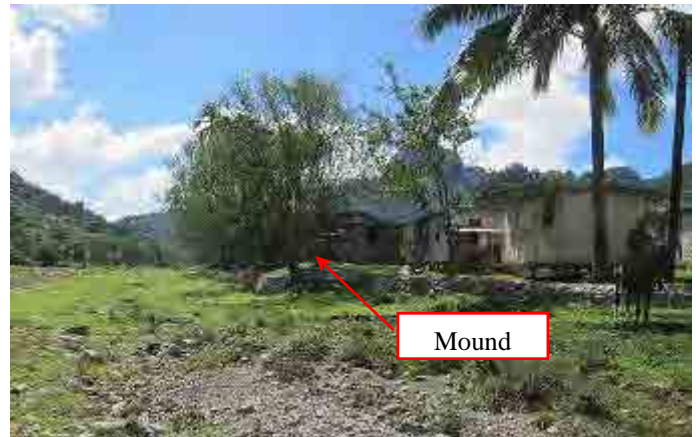
Photo-2 Condition of Wainatava village Top level of mound surrounding the villagers' houses is El.130m. (View from Nakavika River)
