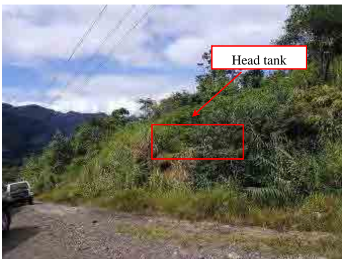
Photo-5 Condition of alternative head tank (View from the access road to Rewasau village))
