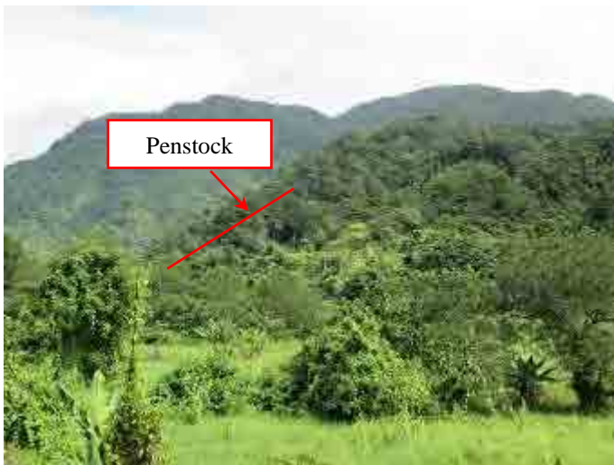
Photo-3 Condition of alternative surge tank and penstock (View from right bank of Waisoi River)
