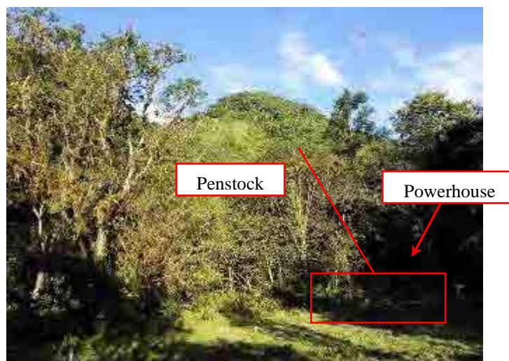
Photo-3 Condition of alternative penstock and powerhouse (View from surrounding powerhouse)
