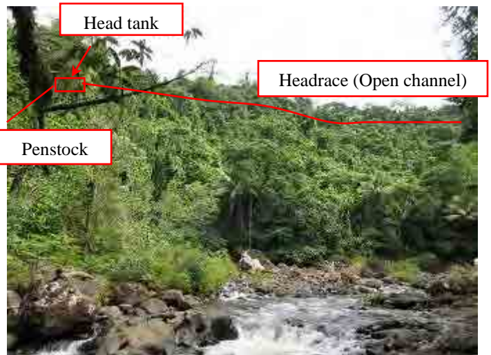
Photo-4 Condition of original Headrace, Head tank, and alternative penstock (View from upstream of left bank on foot path to weir)
