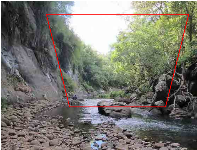
(Photo-2) Condition of alternative dam site for No.2 intake
