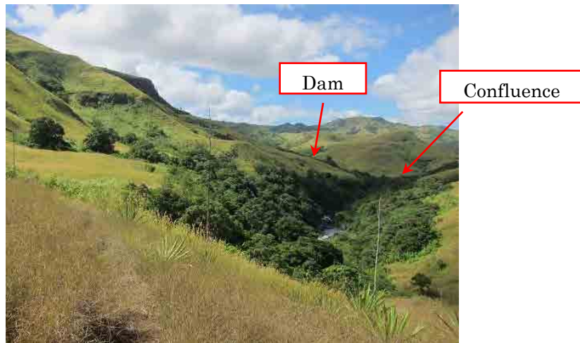
(Photo-5) Condition of alternative dam site for No.2 intake and the confluence of Savatu Creek and Ba River Topographic condition of the right bank of Ba River along the headrace tunnel is characterized gentle slope and steep cliff.
