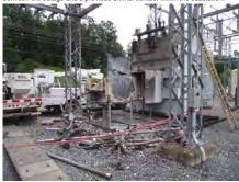
Figure 7-12: Example of damage caused by a snake at a substation Source: http://tdworld.com/substations/protect-your-substations-against-animal-intruders
