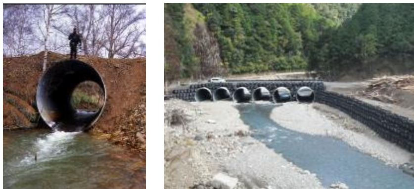
Figure 6.4.1 Temporary Road Utilizing Corrugated Steel Pipes
