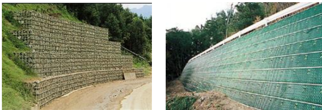
Figure 6.4.2 Examples of Fill Construction Utilizing Gabion Mattress and Geotextile Walls
