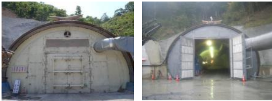
Figure 6.4.3 Installation of Sound-proof Door
