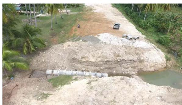
Photo shows the drainage pipe crossing at Sta. 0+120 of MC-3, which is the facility for drainage canal to cross the irrigation canal.
