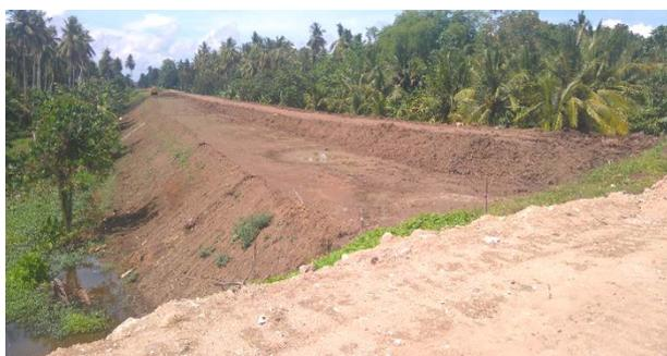
This picture shows portion of MC-3 at the diversion point from RMC-1 EXT-1. The height of canal embankment at this point is about 8.5m to convey the irrigation water to its final section that is 22.8 km away.
