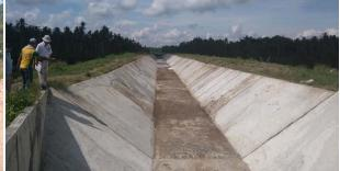
This picture shows portion of MC-3 at the diversion point from RMC-1 EXT-1. The height of canal embankment at this point is about 8.5m to convey the irrigation water to its final section that is 22.8 km away.
