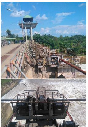
Above pictures show a gate lifting device at spillway. There is no shade to protect them from rain and sunshine, and metal parts of the device rust easily. Actually, in seven devices, the cable is already rusty and broken and the lifting devices are not working properly. The operation of these devices is at risk, hence the operation of the entire dam.
