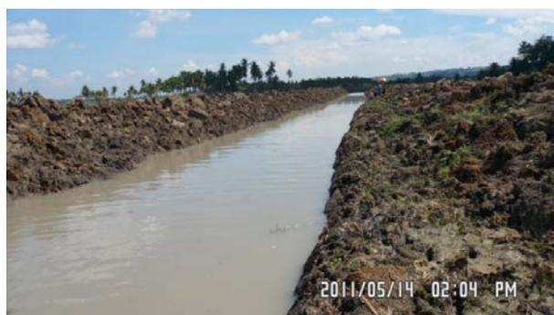
Photo shows the lateral drainage canal (LDC-PR-III) excavated in 2011 to improve the drainage capacity.
