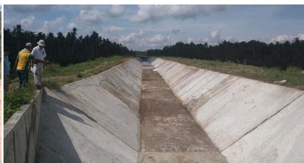
Concrete lining is planned for main canals. Picture shows concrete lining of RMC-1 EXT-1
