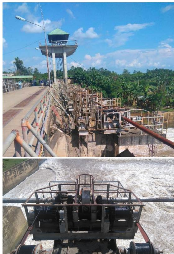
Above pictures show a gate lifting device at spillway. There is no shade to protect them from rain and sunshine, and metal parts of the device rust easily. Actually, in seven devices, the cable is already rusty and broken and the lifting devices are not working properly. The operation of these devices is at risk, hence the operation of the entire dam.
