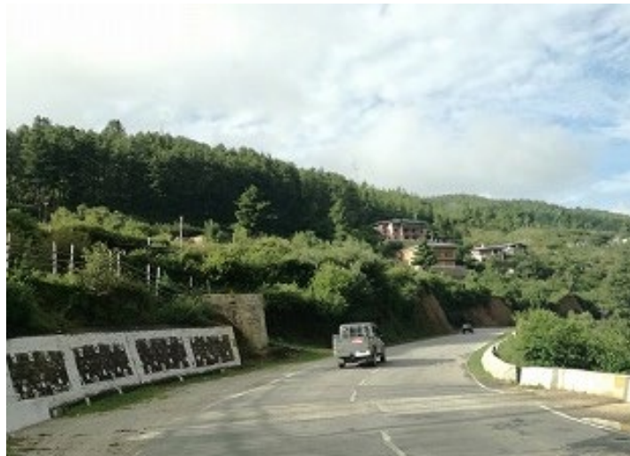
Figure 5.6.14 Retaining Wall on a Road between Thimphu and Paro
