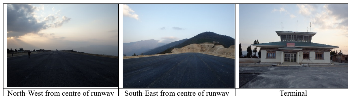
Figure 5.3.8 Yonphula Airport (Under Construction as of 11 April 2017)
