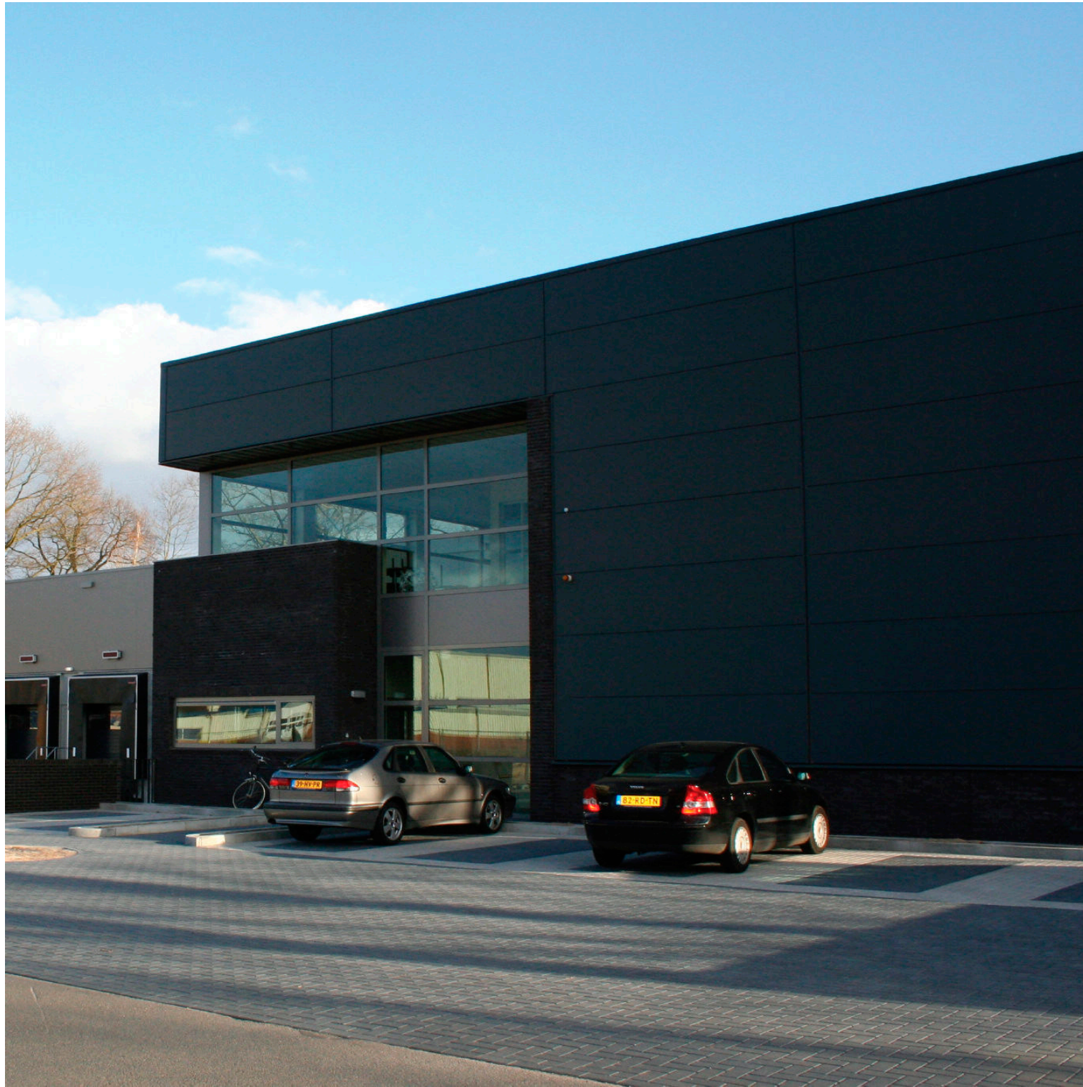
Sandwich Panel- structure made of three layers: a low density core, and a thin skin-layer bonded to each other
