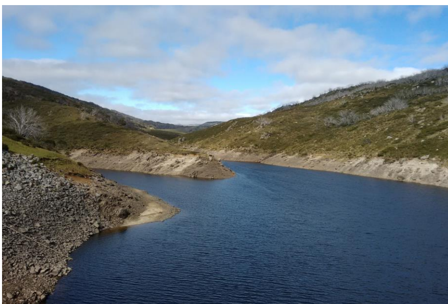
Figure 24: Dams built for the Snowy Hydro scheme resulted in peatland loss (Photo: Anne Murray)
