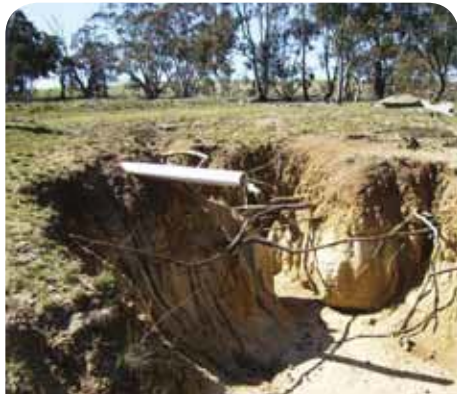
Figure 4.5: This State 2 woodland was already susceptible to erosion, but incorrect placement of this runoff diversion pipe (middle) probably made it much worse. The pipe was allowed to discharge water at a height, displacing large amounts of soil.
