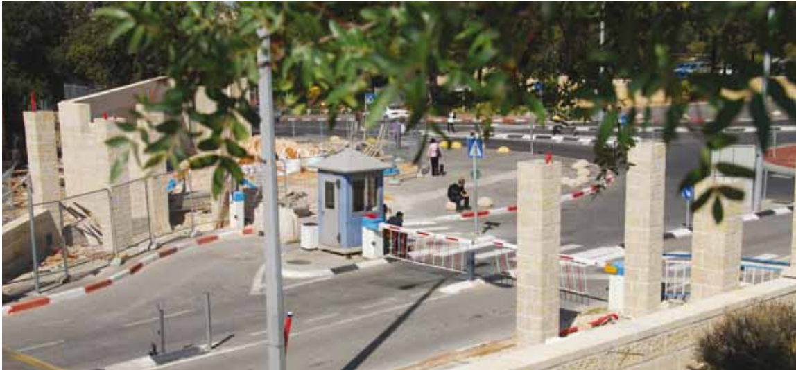
Construction of the new main entrance to the Mount Scopus campus
