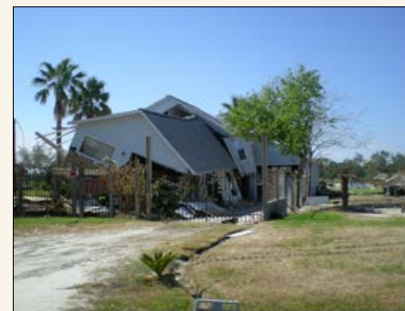
Hurricane Ike Impact. South Texas 2008
