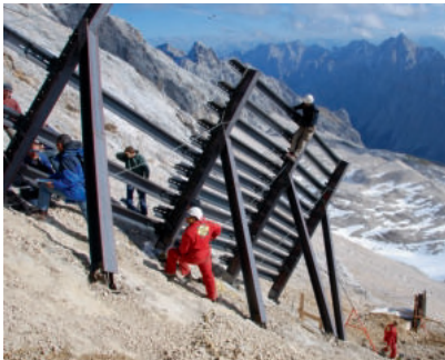
Fig. 23: View of the construction site for the integrated rockfall and avalanche protection system for the high-altitude research station UFS (see also Fig. 25)
