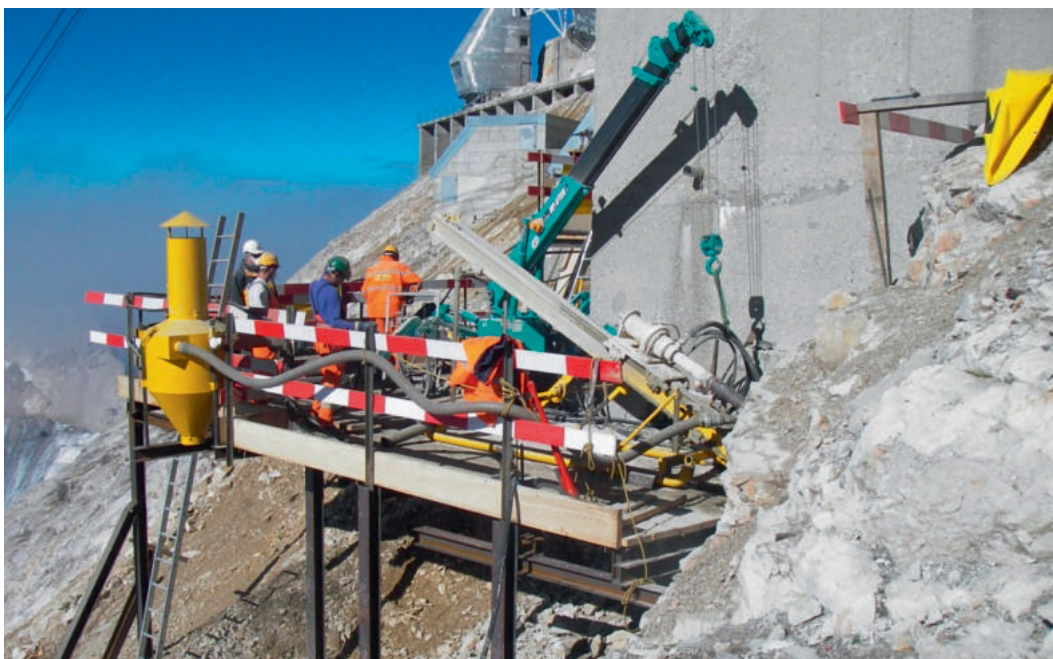
Fig. 2: Platform with drill carriage, minicrane and dust protection filter.
