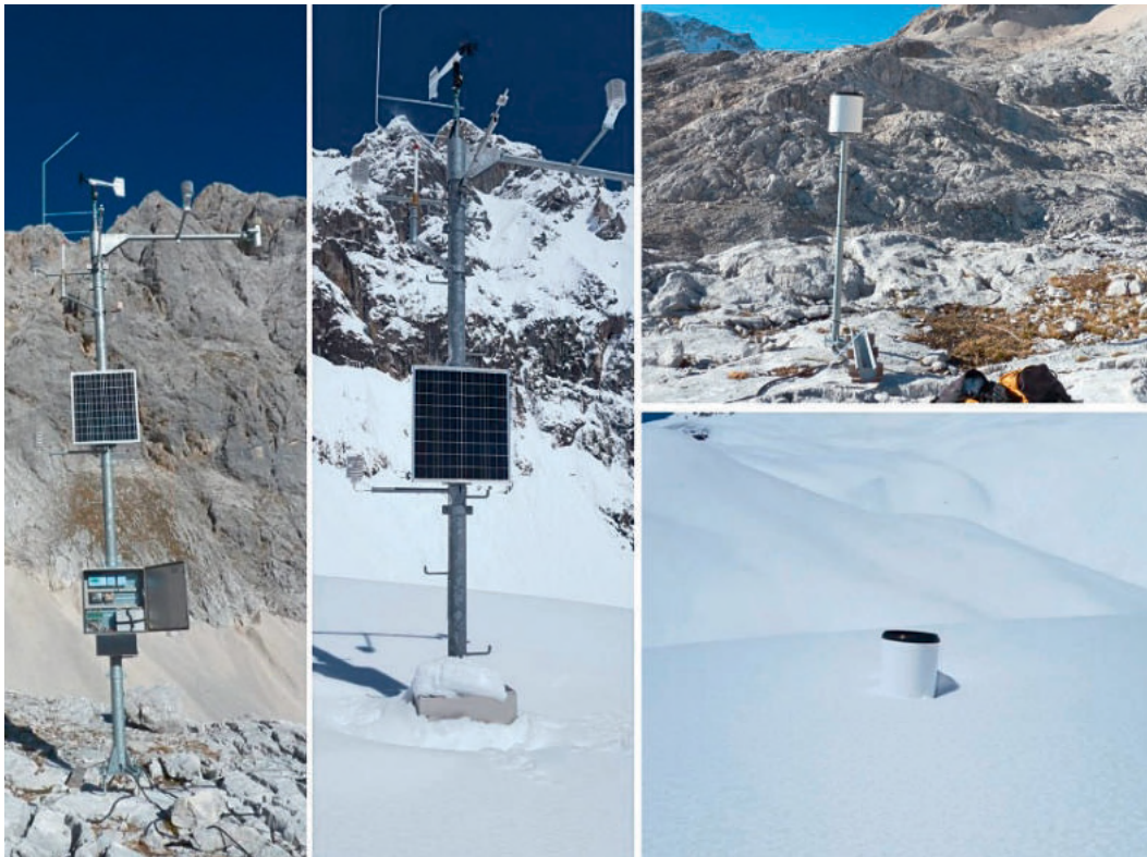
Fig. 4: Summer and winter aspect of a meteorological station in the RCZ.
