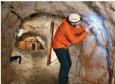
Fig. 24: Permafrost measuring system, installed in the remaining summit tunnel between the UFS and the former terminus of the "Austrian Zugspitze Cable Car"
