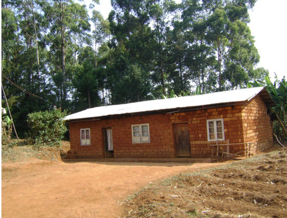
Plate 18: The Predominant Mud-bricks constructed House in Oku
