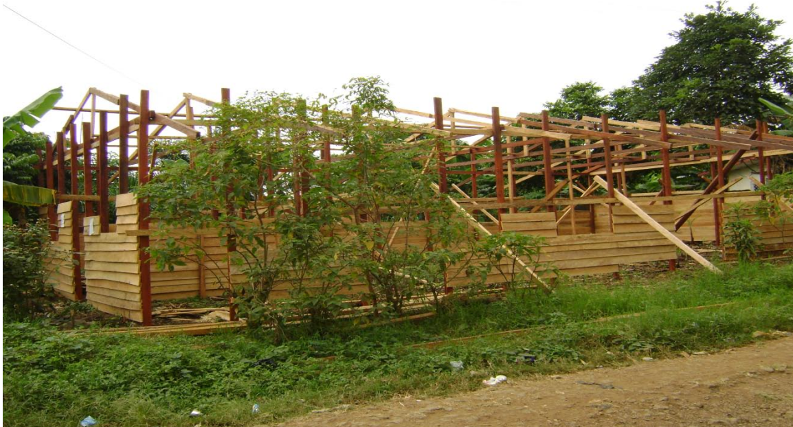
Plate 16: A Wooden House ( Karaboat ) under construction in Bonakanda, Buea
