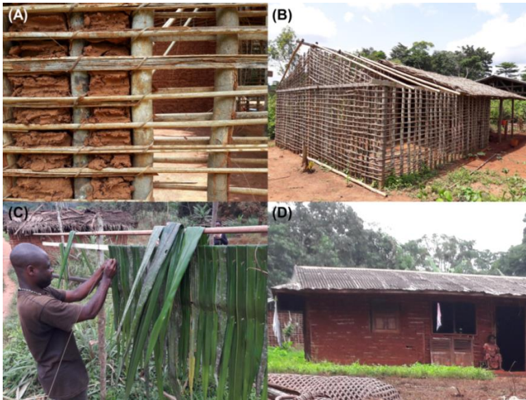
Figure 4.3: Traditional house type considered for the estimation of timber use in the integrated assessment of ecosystem services use in three villages (Dja area, southeastern Cameroon). (A, B) Traditional house structure. (C) Making of straw roof. (D) Roof plate.
