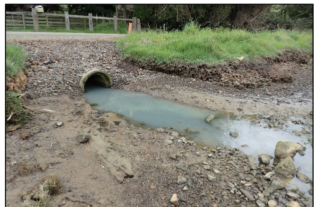
Localised freshwater input from an under-road culvert
