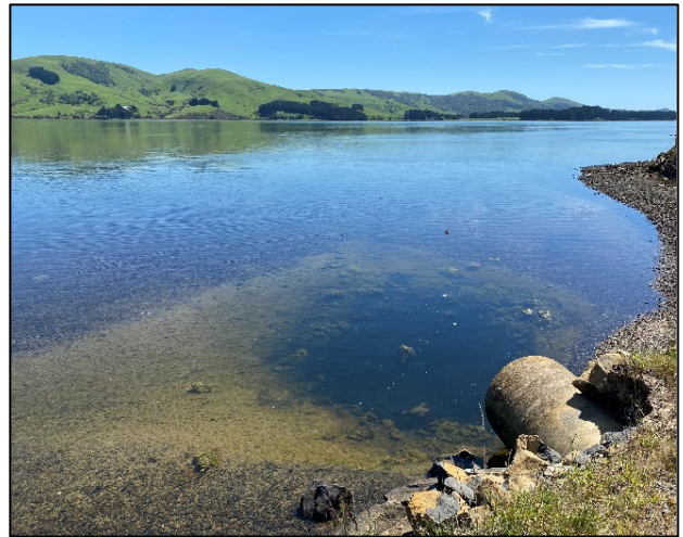
Low oxygen sediment directly below drain outlet
