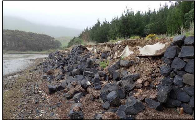
Artificial boulder field and gravel field on road margin (top) and eroding artificial boulder field (bottom)
