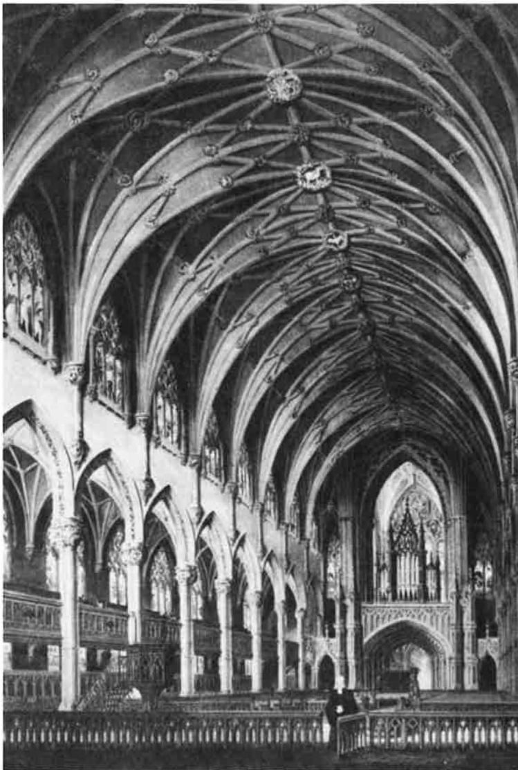
The case of Henry Crabb's three-manual organ of 1845 remained in Holy Trinity Church, Brooklyn, surviving work done on the organ by Johnson and the 1873 rebuilding by Roosevelt, but was replaced when the Hutchings arrived in 1899. This image of the interior is from a watercolor.
