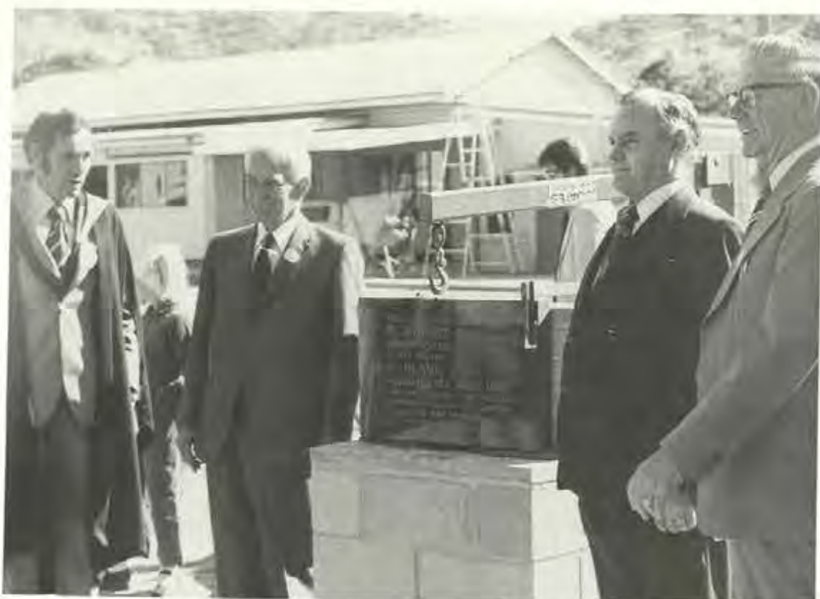
LAYING THE FOUNDATION STONE OF THE ENGLISH DEPARTMENT JUNE 23, 1979
