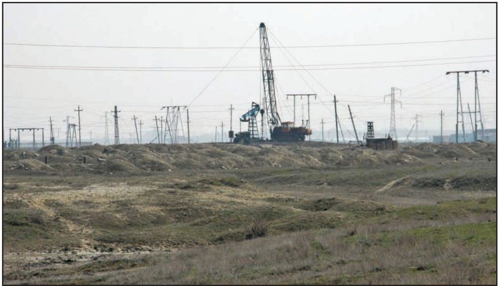
Plate 11. A view through the Besh Barmag bottleneck showing parts of an oil production plant crossed by several power lines. Collisions with these may pose a threat to migrating birds, but as yet no detailed investigations have been conducted. Furthermore, this picture shows the extent of infrastructural development in the bottleneck area and since the construction of the near highway along the coast, which crosses the counting station, it becomes clear that space for conducting bird migration counts is getting more and more reduced. Besh Barmag, Azerbaijan, 21 March 2012. © Michael Heiss
