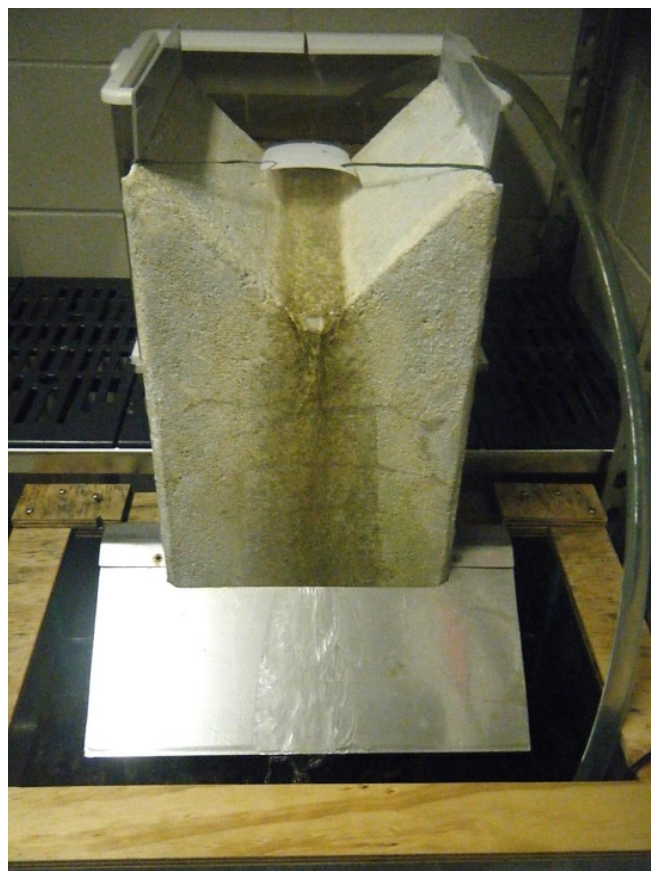
Fig. 3.2 Alloy barrier installed on the concrete weir (photo: Josh Tabak)
