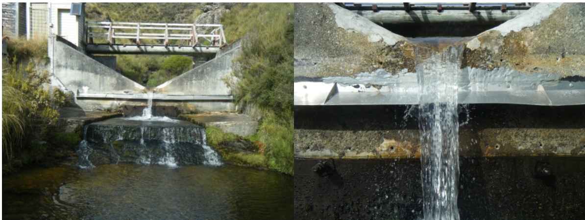
Fig. 4.3 A new perched migration barrier design to stop climbing juvenile kōaro (photo: Josh Tabak)
