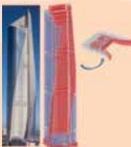
Fig. 2. Finite element model of the Al-Hamra Tower
